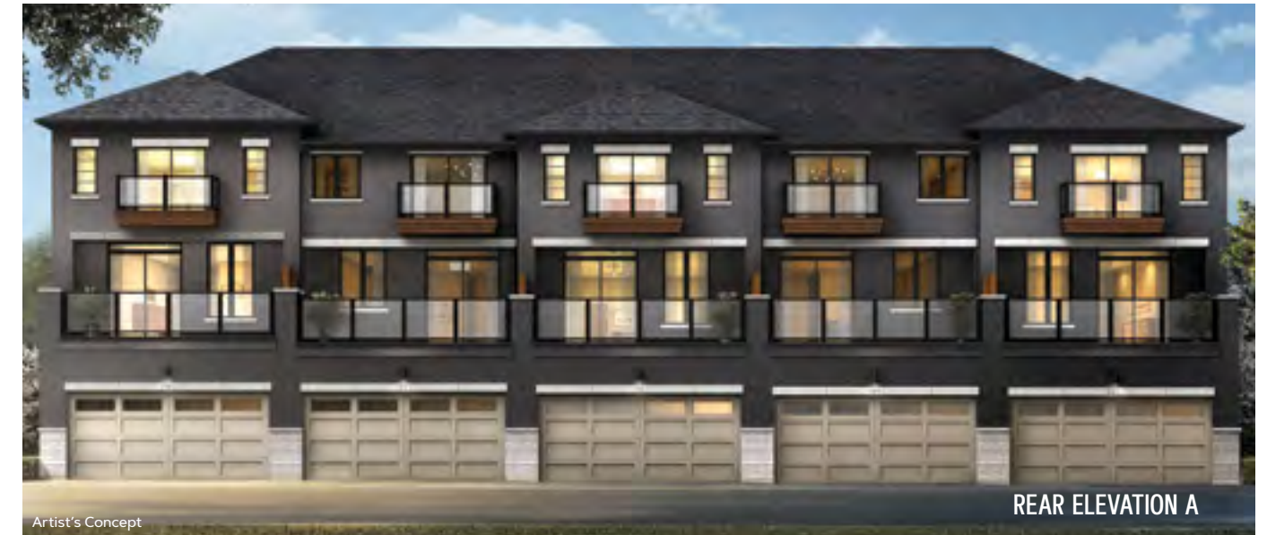
Artist's Concept REAR ELEVATION A RL-3 CORNER RL-1 RL-2 RL-1 RL-3 CORNER
